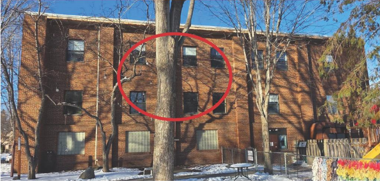
This photo of the south wall of the church shows the area where water has entered the building walls and is affecting the rooms on the second and third floors.
